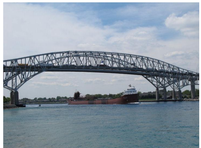
St Clair River under the Bluewater Bridge.
